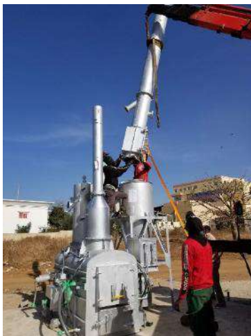
Senegal Installation of incinerator
