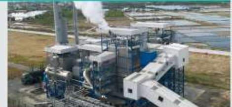
Biomass Boiler (Vietnam) Marubeni Corporation
