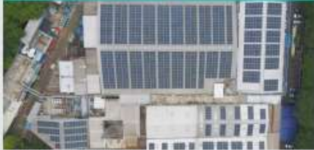
Solar Power (Indonesia) Alamport Inc.
