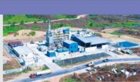
Waste to Energy Plant (Myanmar) JFE Engineering Corporation
