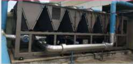
Air Cooled Chiller (Vietnam) Hitachi-Johnson Controls Air Conditioning, Inc.
