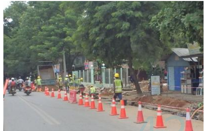
Back Filling & Road Restoration
