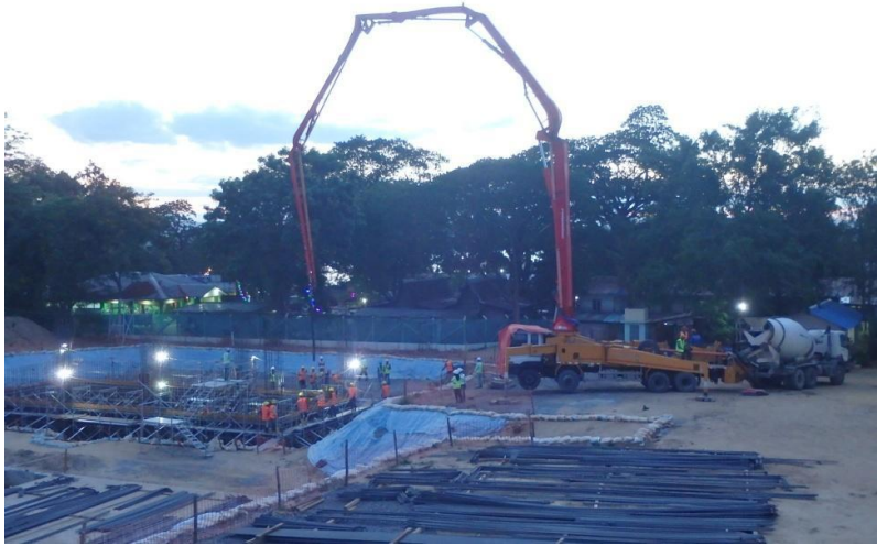
Concrete Casting for Wall of Pump Pit
