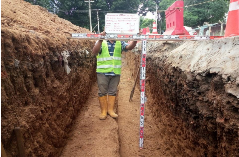
Inspection for Depth of Pipe Bed
