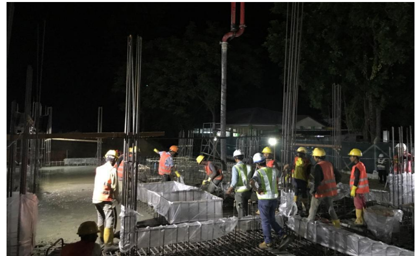
Concrete Casting at Distribution Pump Station
