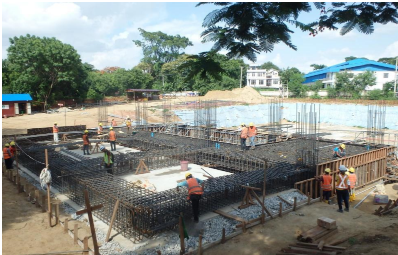
Reinforcing Bar & Form Installation at Distribution Pump Station
