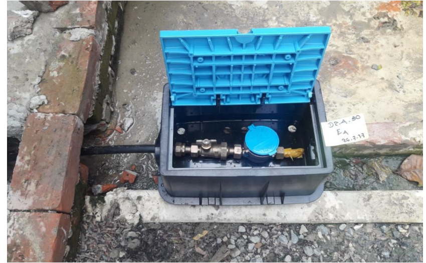
Water Meter Installation
