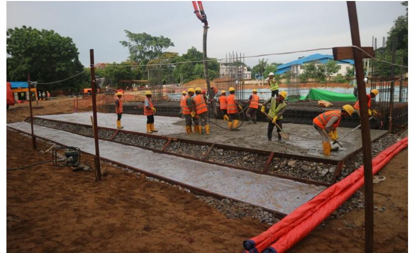
Lean Concrete for Chlorination Room
