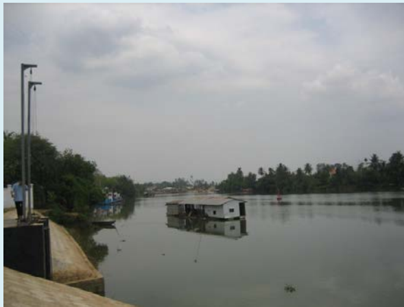
Surface water intake point
