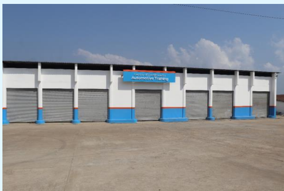
Post rehabilitation of Automotive Center
