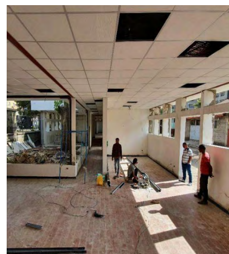
Creative Hub finishing works undergoing
