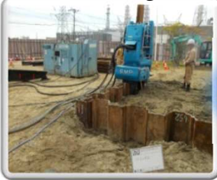
Earth retaining work
