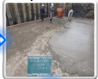
Primary concrete work
