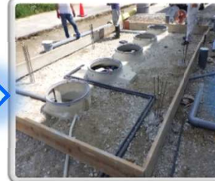
Air piping work
