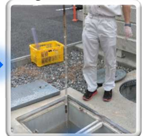
Sludge thickness check
