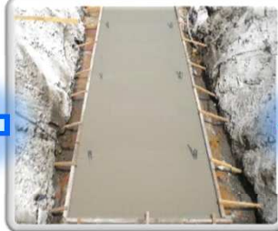
Base concrete work
