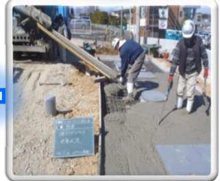
Slab concrete work
