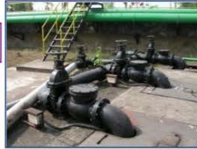
PUMPS to Aeration Tank
