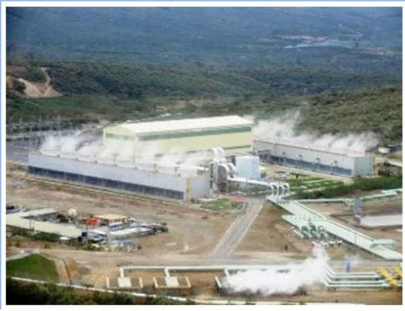
Olkaria IV Geothermal Power Plant, Kenya (Photo: Toyota Tsusho)
