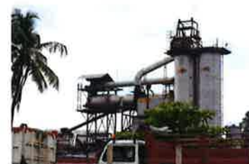
Picture 2 Asphalt regeneration plant
