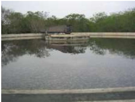
PRIMARY SEDIMENTATION TANK
