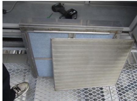
Removal of grease filter
