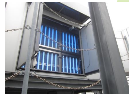
Removal of photocatalytic filter
