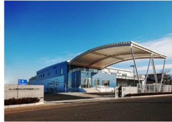
Saitama "N school central kitchen"
