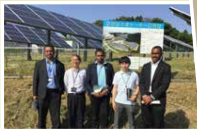
The Fijian Delegate visited a solar power plant.
