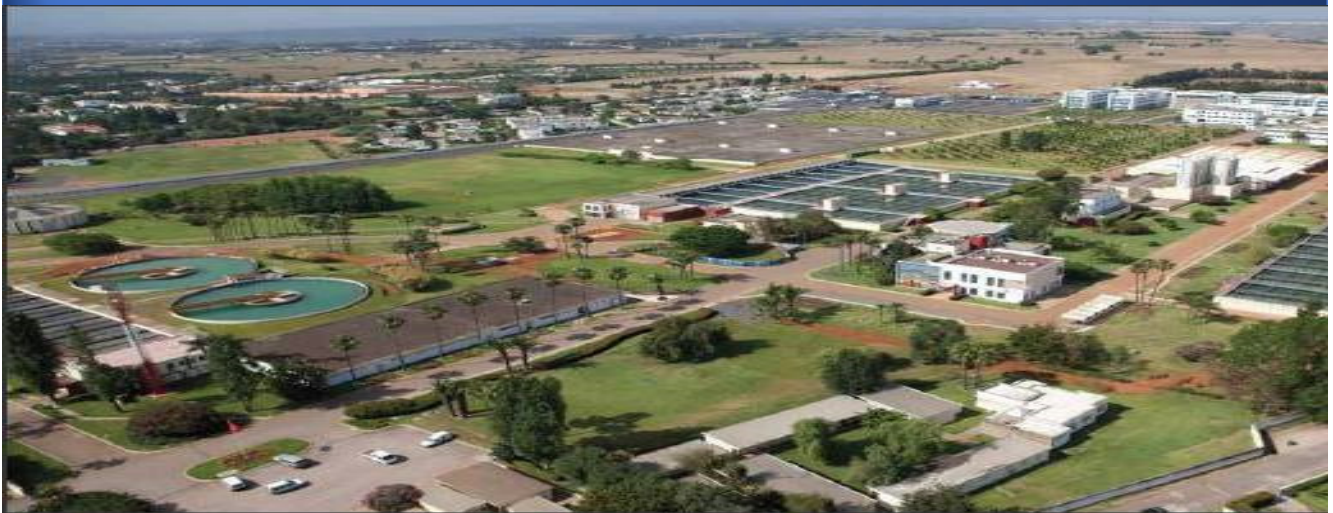
Bouregreg treatment plant (10 m 3 /s) ONEE - RABAT
