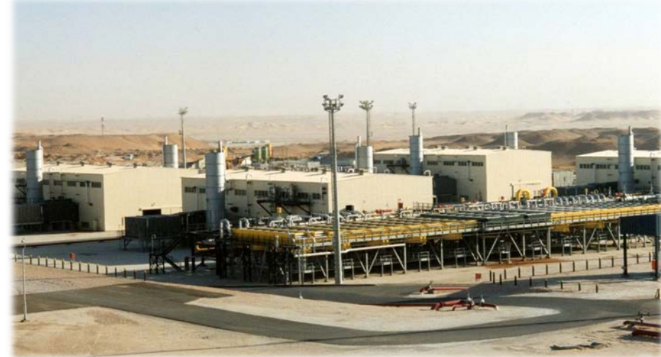
HASSI MESSOUD COMPRESSOR STATION (1987-1990)
