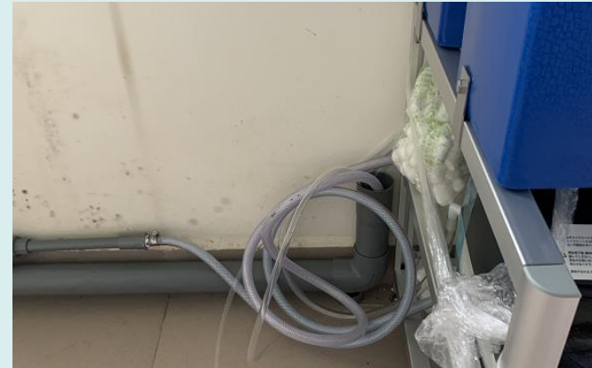
Preparation of drain
