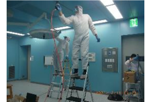
Mongolia Application of photocatalyst coating at the hospital
