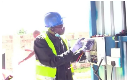
Kenya On-site assembly and installation of a medical waste incinerator
