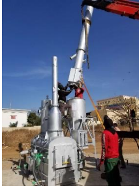
Senegal Installation of incinerator
