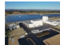
Power to Gas
