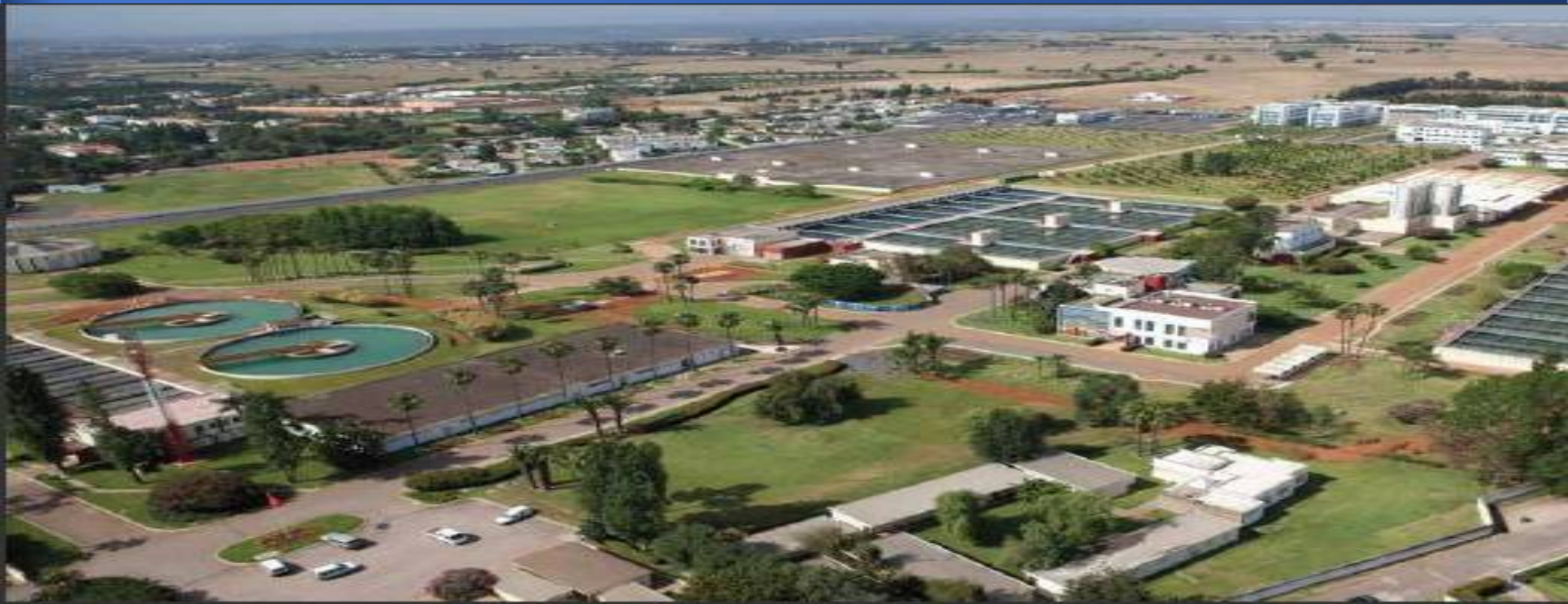
Bouregreg treatment plant (10 m 3 /s) ONEE - RABAT
