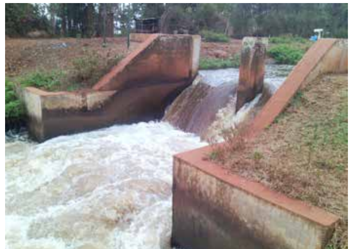
Photo after and before the installation of the 10kW ULHMHP system at an irrigation canal close to Kiuria village in Mwea (Kenya)
