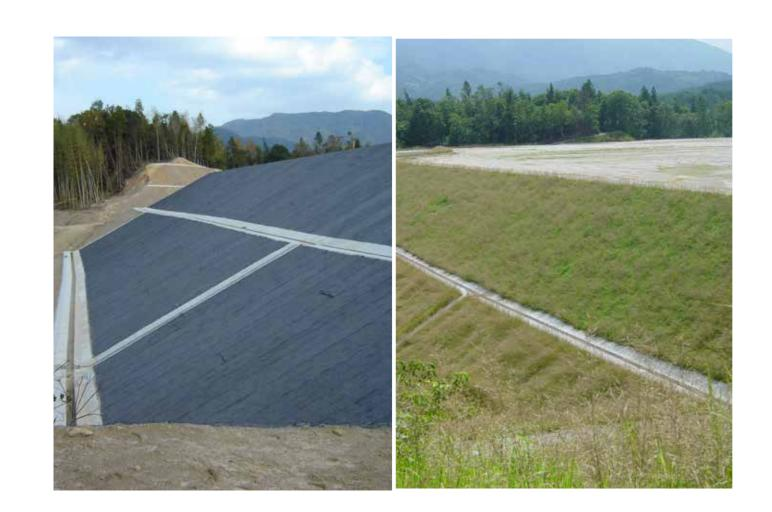
The multifunctional filter is a greening mat that prevents soil erosion and is found at construction sites related to infrastructure such as roads, disaster recovery work, and natural resource extraction.
