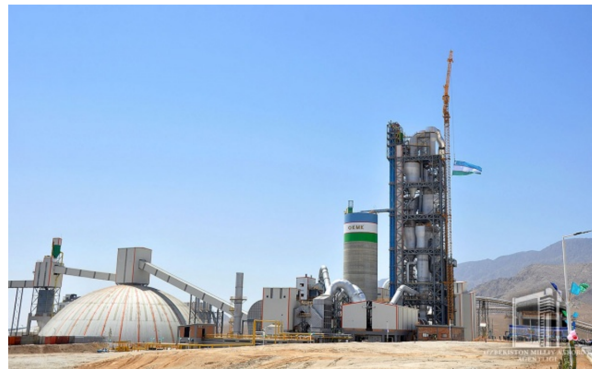
Cement production plant for 1 mln. tons a year. Established on Russian investment. Total investment over 39 mln.USD
