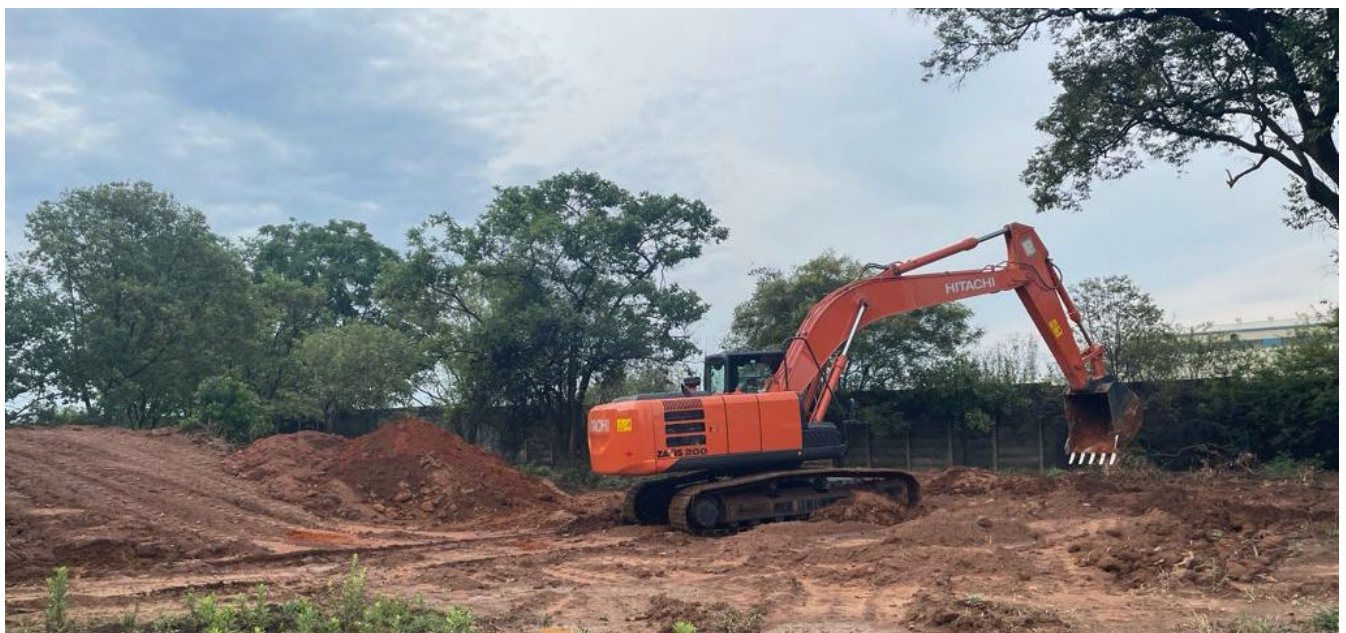
Trench crossing exercises
