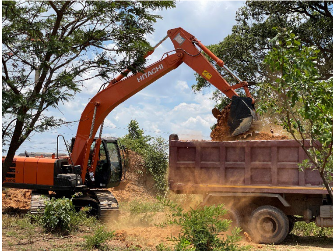
Loading operation in a tipper truck
