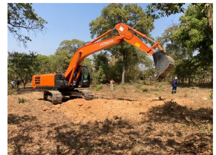
Excavator positioning and coordination
