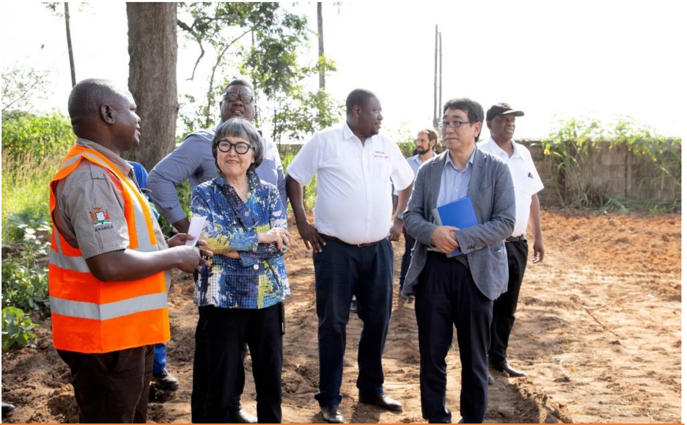
THE VISITING DELEGATION TOURING THE TRAINING AREA AND PROPOSED WORKSHOP CONSTRUCTION SITE AT KVTC.
