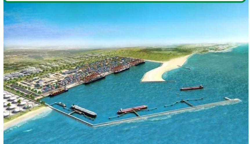
Lekki Port – Nigeria : $1.5B
