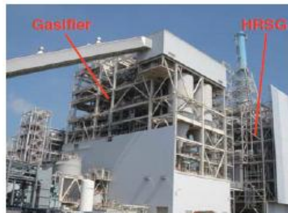
Nakoso IGCC demonstration plant 250 MW operation started in 2007
