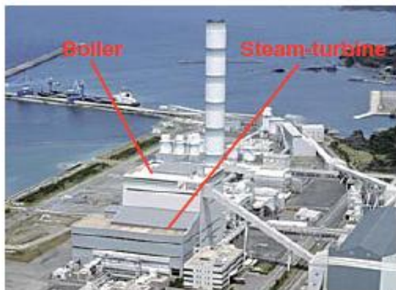
Misumi coal-fired power plant 1000 MW, 24.5 MPa \times 600 ^{\circ} C/600 ^{\circ} C operation started in 1998
