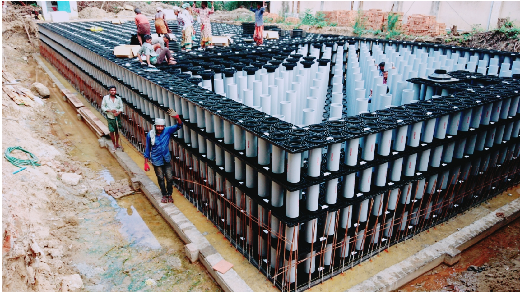
Construction of universal underground storage system for Tamil Nadu, India
