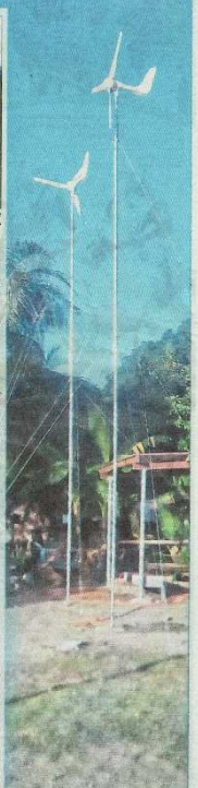
Wind turbines installed in Brooker Island.
