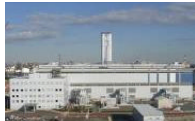
Steam supply source (TEPCO Kawasaki Thermal Power Station) – generating efficiency of 59%, the world's highest level
