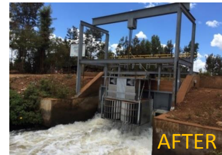
Before & After installation of the ULH-MHP at Mwea Irrigation Canal in Kenya
