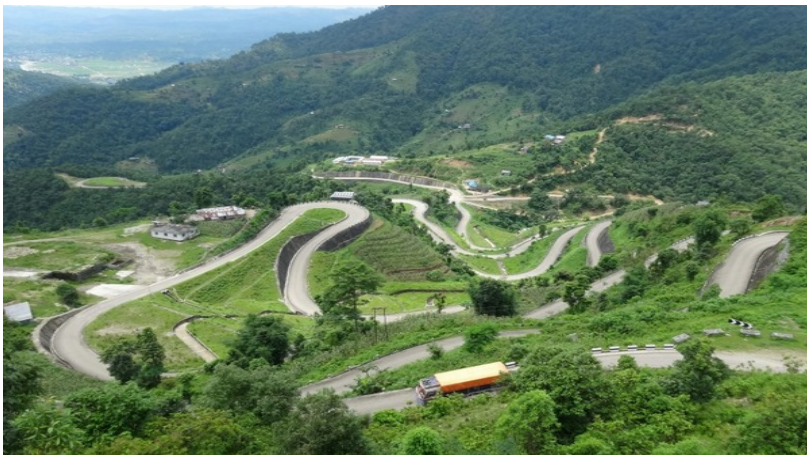
Sindhuli Road (2015) BP Highway.
