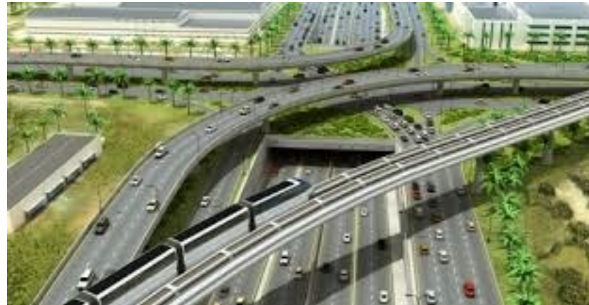
Roads, railways and interchanges on BOT
